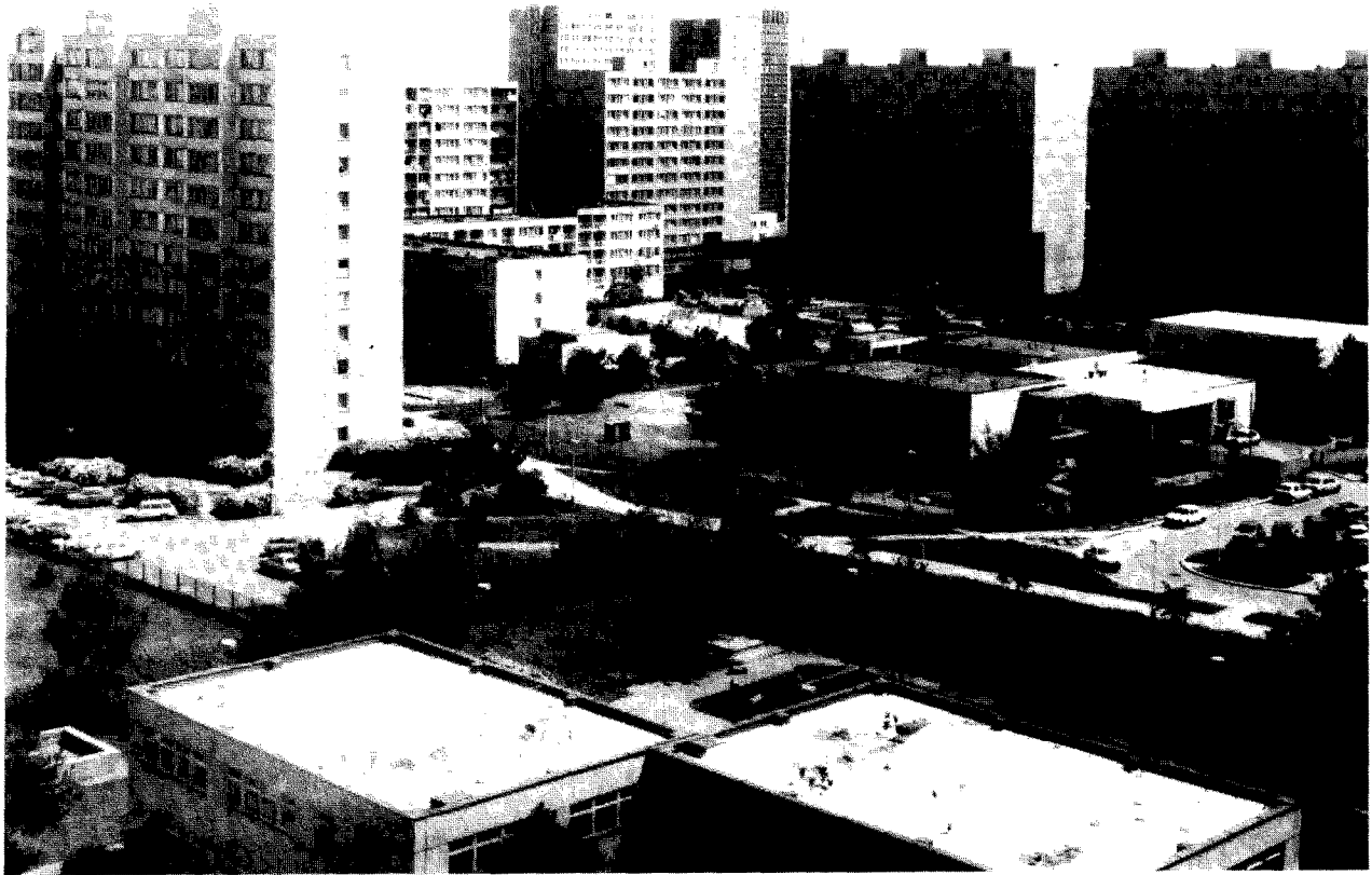
Figure 4. The housing estate built in the 1970s: South Town.
