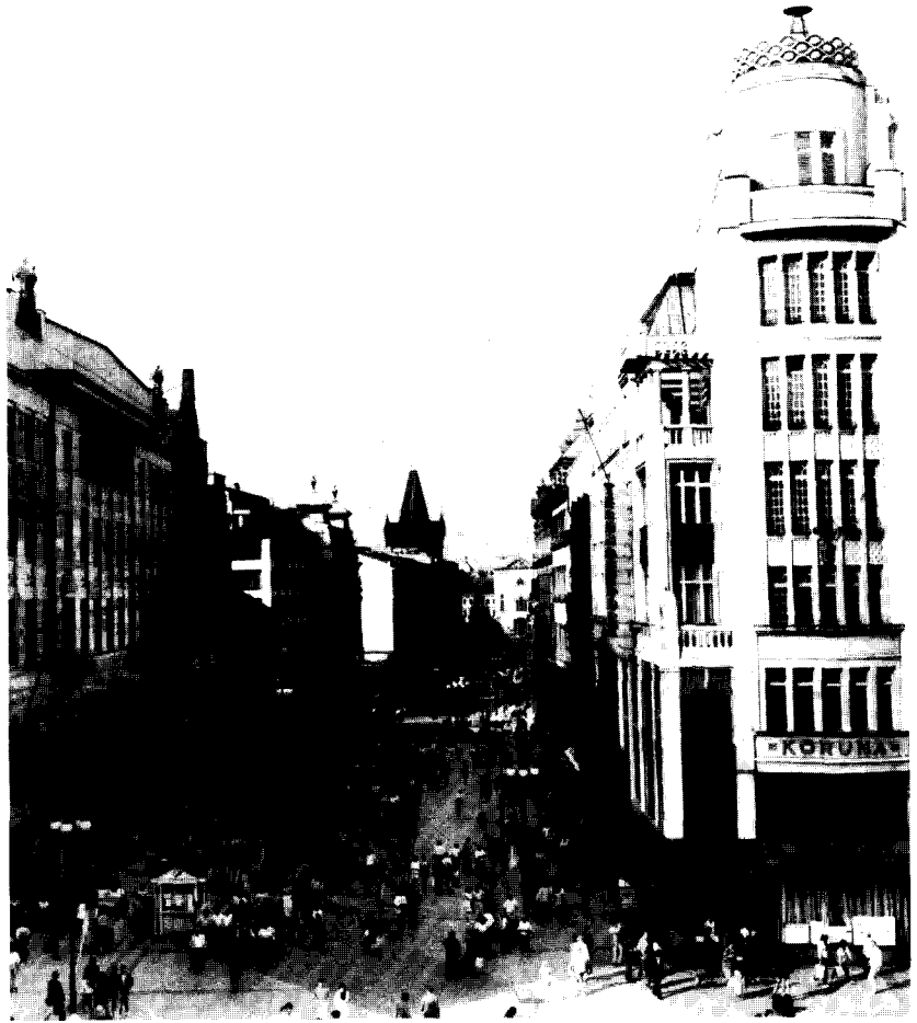
Figure 5. Pedestrian zone in the CBD.
