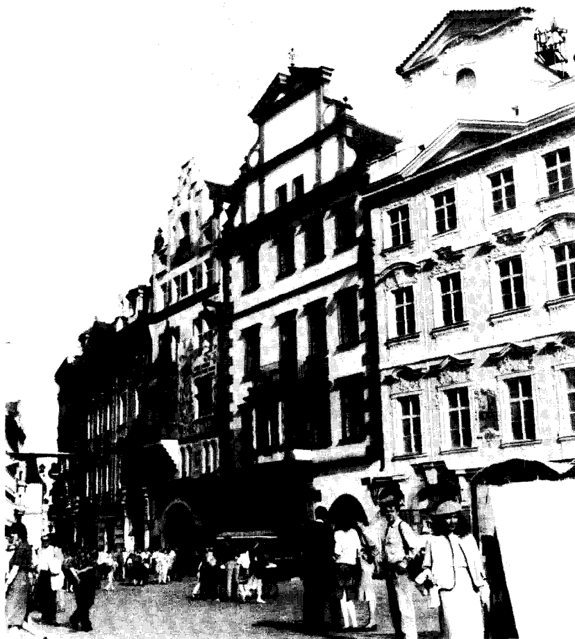
Figure 6. Rehabilitation of the mediaeval houses in the Old Town Square.
