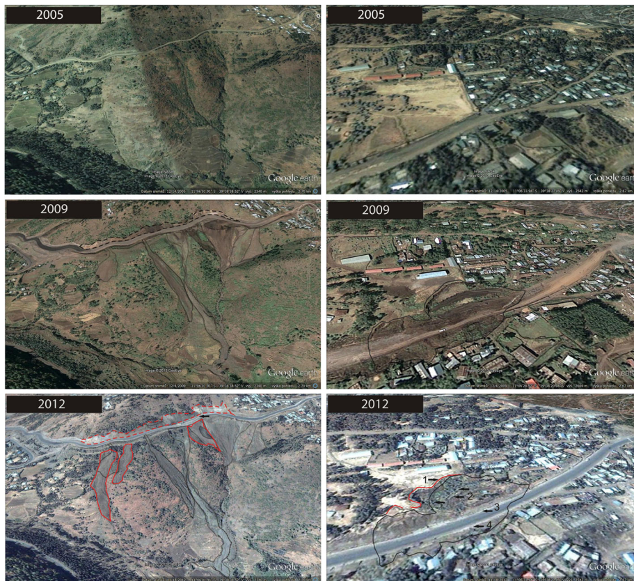
Fig. 4 Comparison of the noticeable development of the studied landslide areas (Menbere Tshay area—right, Dessie–Kombolcha road—left) in the years 2005–2009–2012; the first landslide events were caused by the construction of a new asphalt road leading to Dessie town. Numbers in the Menbere Tshay area (2012) indicate the remedial works RW1, 2, 3 and 4
