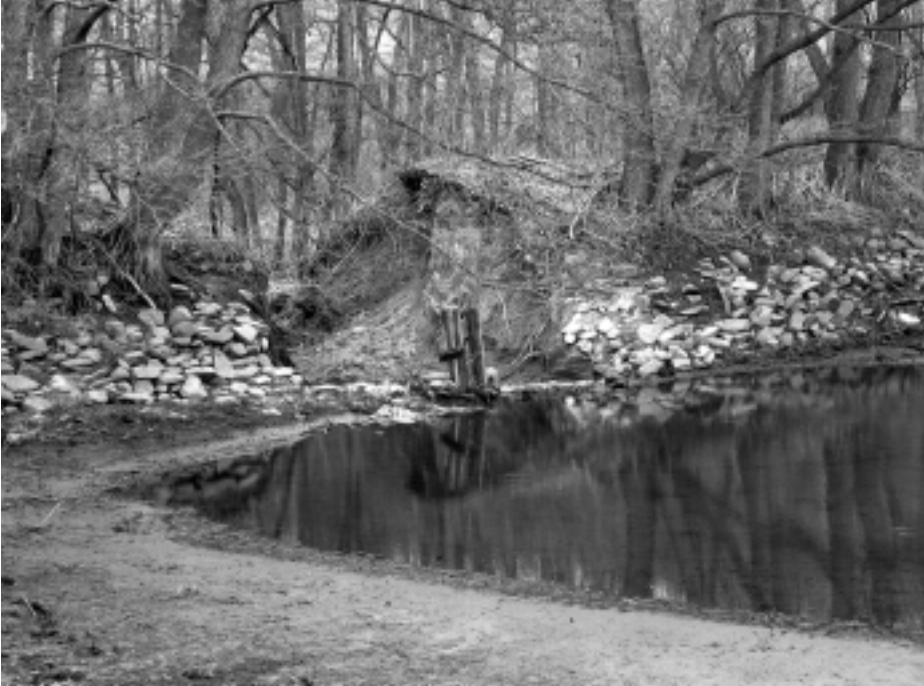
Fig. 1: The Blažňov pond after the dam breach. The depth of the rest of water in the pond was 0.3 m
