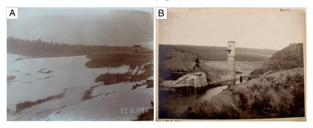
**Fig. 4.** Upstream view of the Desná dam before (A) and after (B) the dam failure. Source: Archive of the Jablonec nad Nisou, Court reports.
