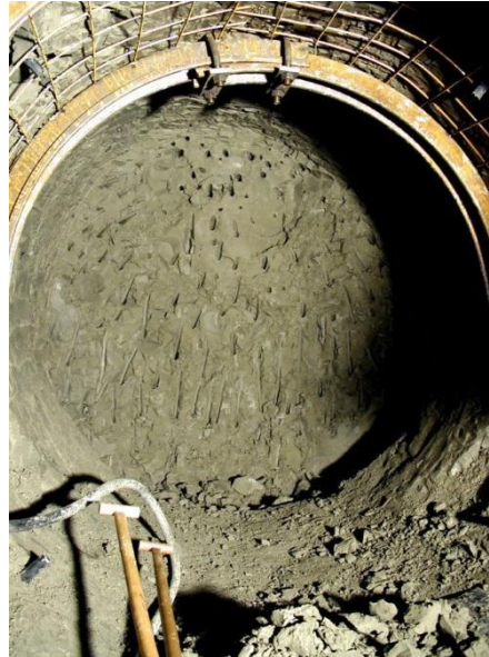
308 Fig. 9. Lining with the offset of 50 mm from the soil (adit R2; photo by J. Pavlík).
