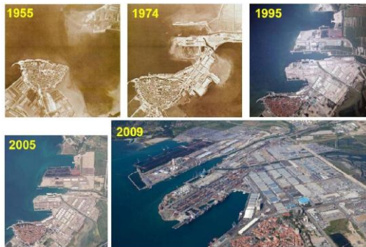
Figure 2. History of development of the Koper town and harbour, demonstrating extensive use of land reclamation (after Logar 2009).
