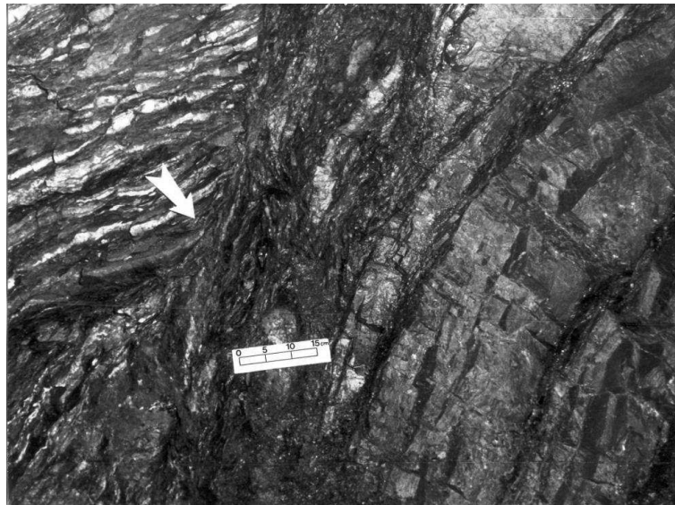
Figure 4: A photography of a small shear zone in the tunnel Mrázovka [3].
